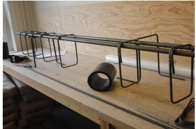
Fig.No:8.3 Reinforcement for beam
