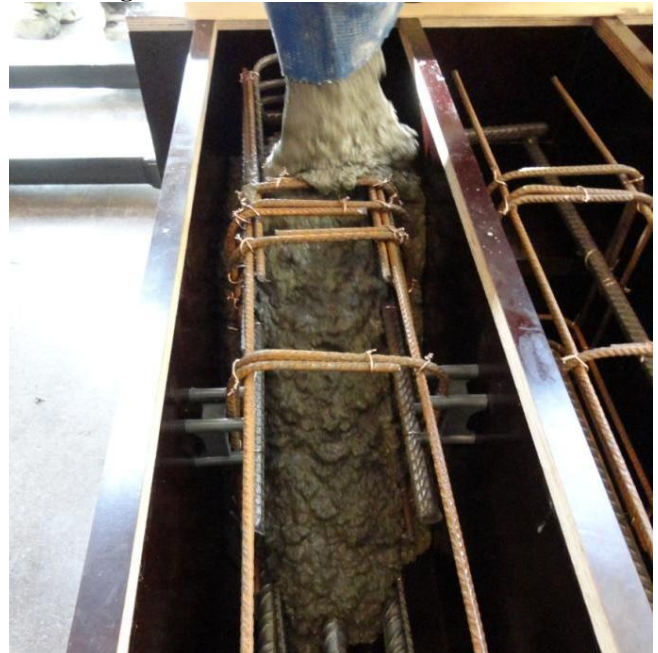
Fig.No:8.4 The Beam casting process
